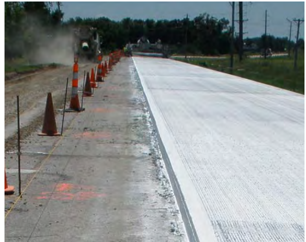
The Oak Crest Hill Road $1.845 million stimulus job is a concrete overlay that covered two lanes and spanned nearly 5.5 miles from start to finish. The road was widened to provide an extra lane for bicyclists.
